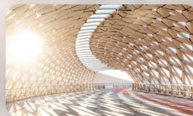
Atyrau Bridge Astana
